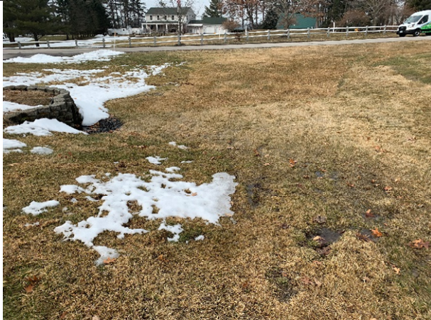
29 Gundalow - 1 (Drainage Area)
